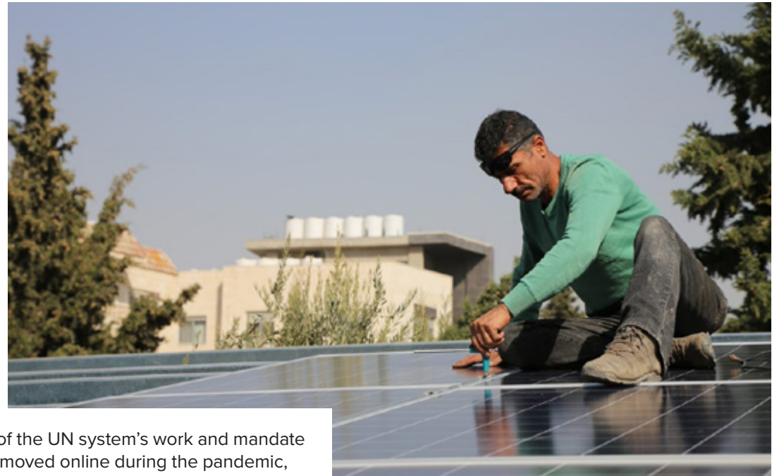
Installation of 760 solar panels in Jordan. Credit: WFP/Dina El-Kassaby
